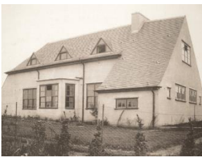
Figure 60 - Back side of the house (photo of 2010)
