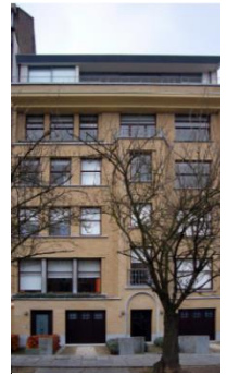
Figure 50 – Personal residence of Yvan Blomme
