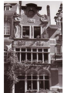
Figure 18 - Personal residence of E. Linssens
