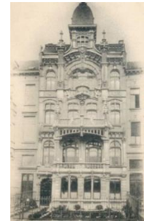
Figure 13 - Personal residence of Antoine Aulbur
