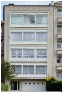
Figure 31 - Personal residence of Henri Montois
